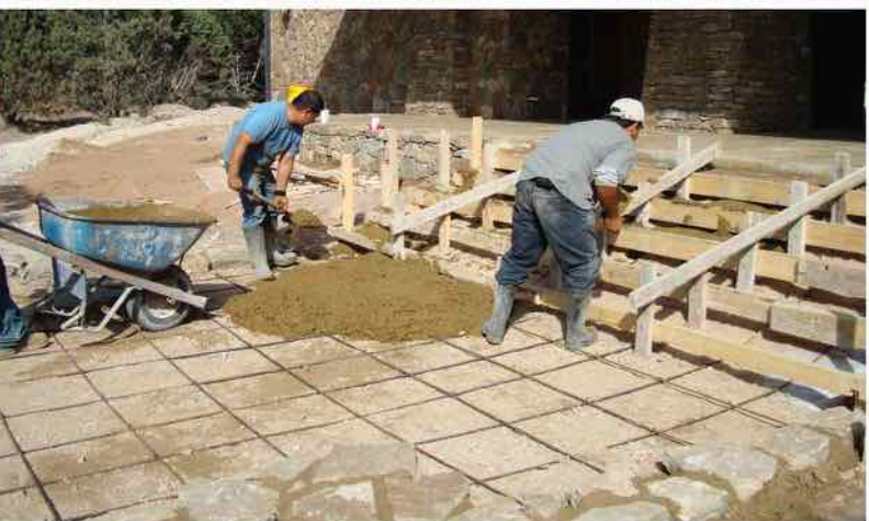
front walkway "color test" concrete pour
