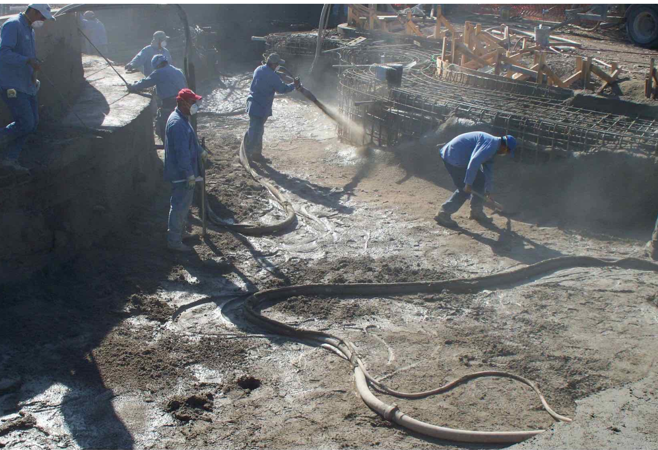
5 gunite crews coordinated
